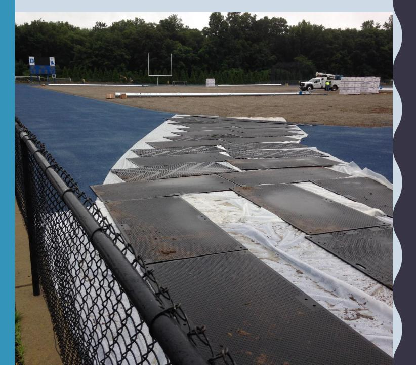
This is the protection of the track so the crane can cross without causing structural damage.
