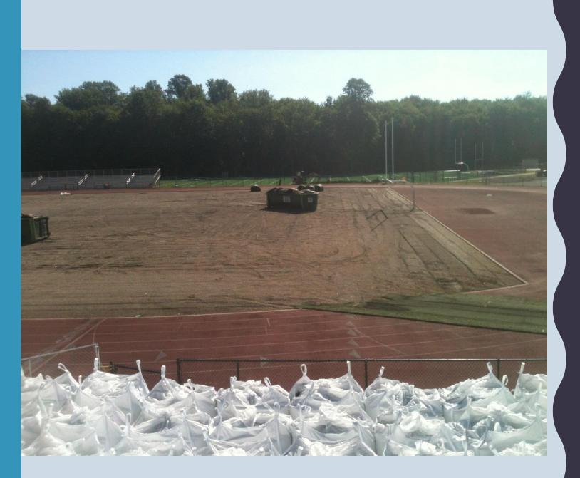
The recycled crumb rubber is temporarily stored in the canvas bags, to be used for the construction of the new field. The dumpsters are used to haul away the old turf, which is in rolls. That material will be recycled by Field Turf.
