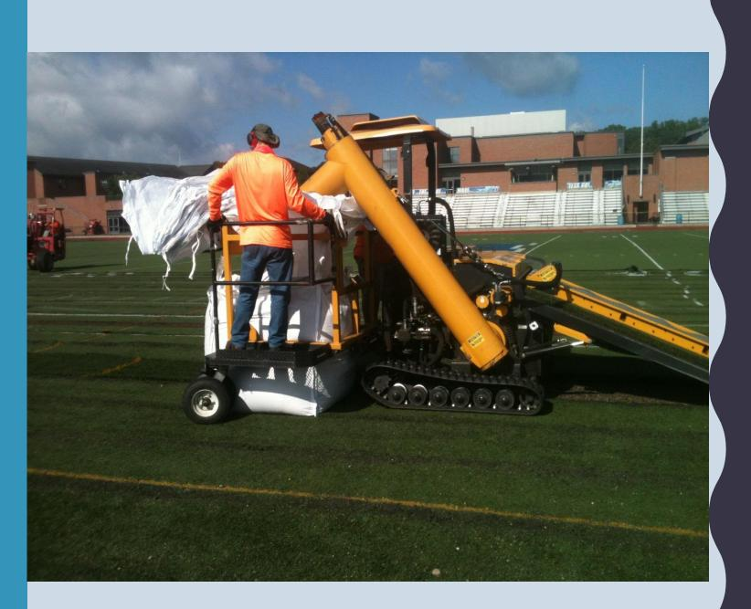
After the turf is sliced, a machine is used to recycle the crumb rubber.
