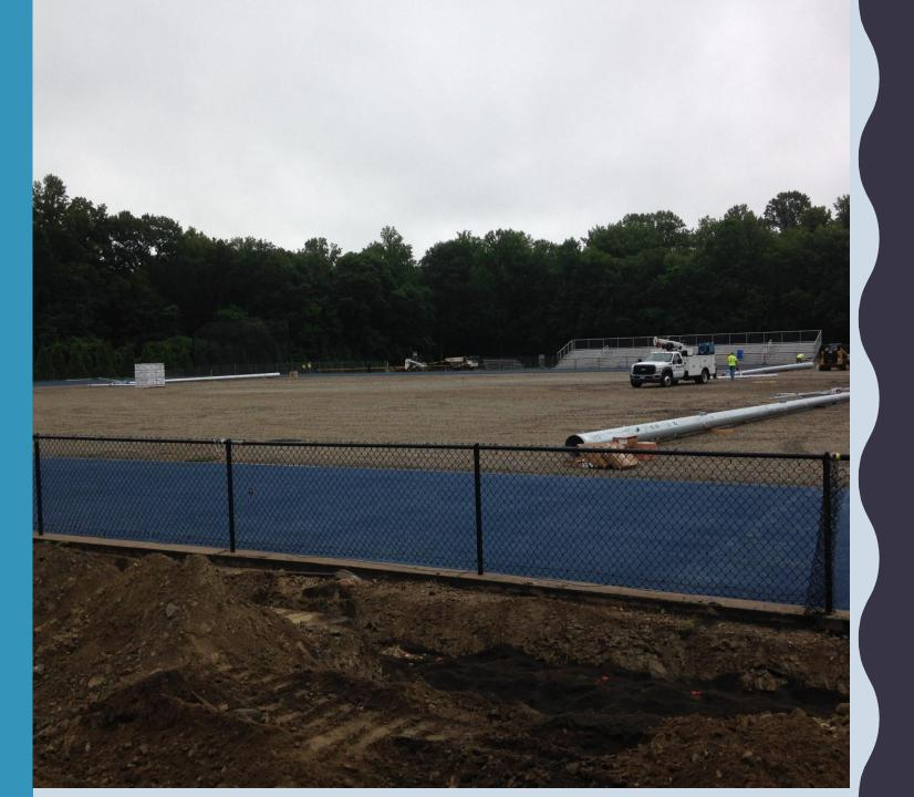
These are the assembled light poles, the day before installation. A crane was used to place them on the foundations.
