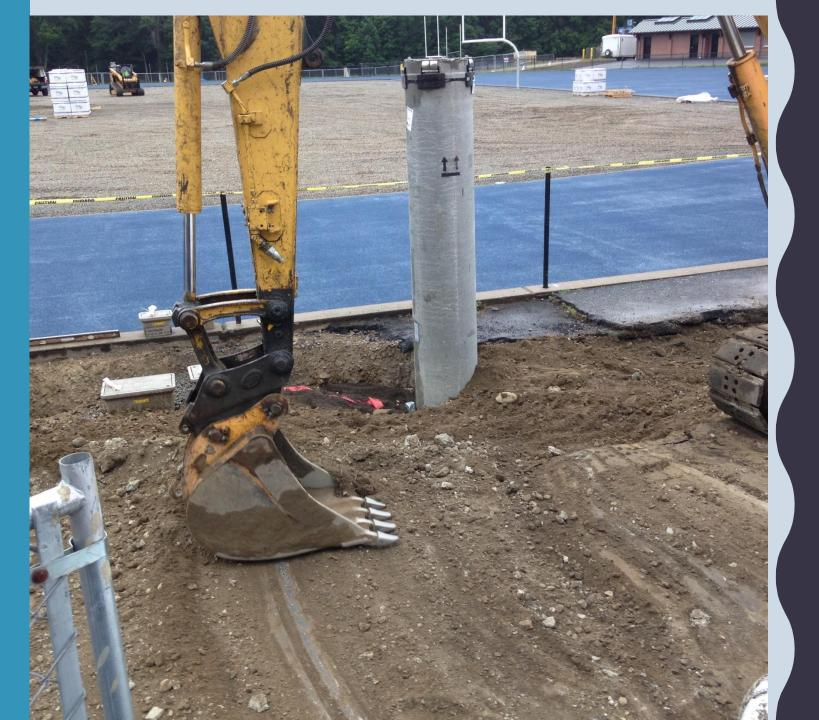
Here is one of the bases for the light poles. The pole is 8 ft. above grade and 14-16 feet below grade. The band around the top is the grounding.
