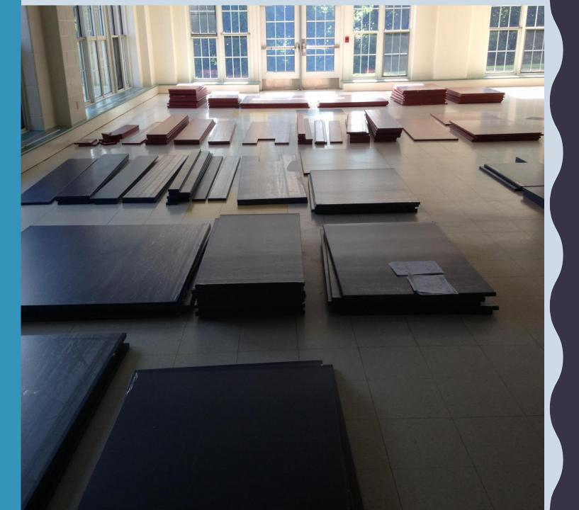
These are the bathroom partitions sorted out by color and location, prior to the installation.
