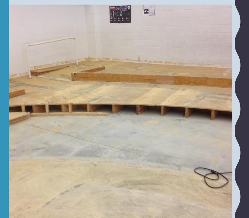
We removed the carpeting and raised floor in the band room at Middlesex. New carpeting will be installed during the last week of August.
